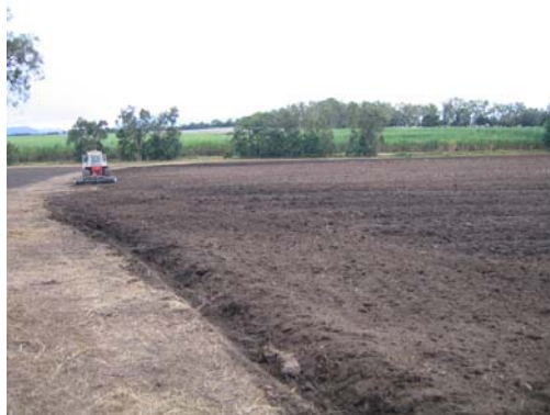
Figure 7 Cultivation of the entire block occurred on 7 June 2006 using off-set discs.
