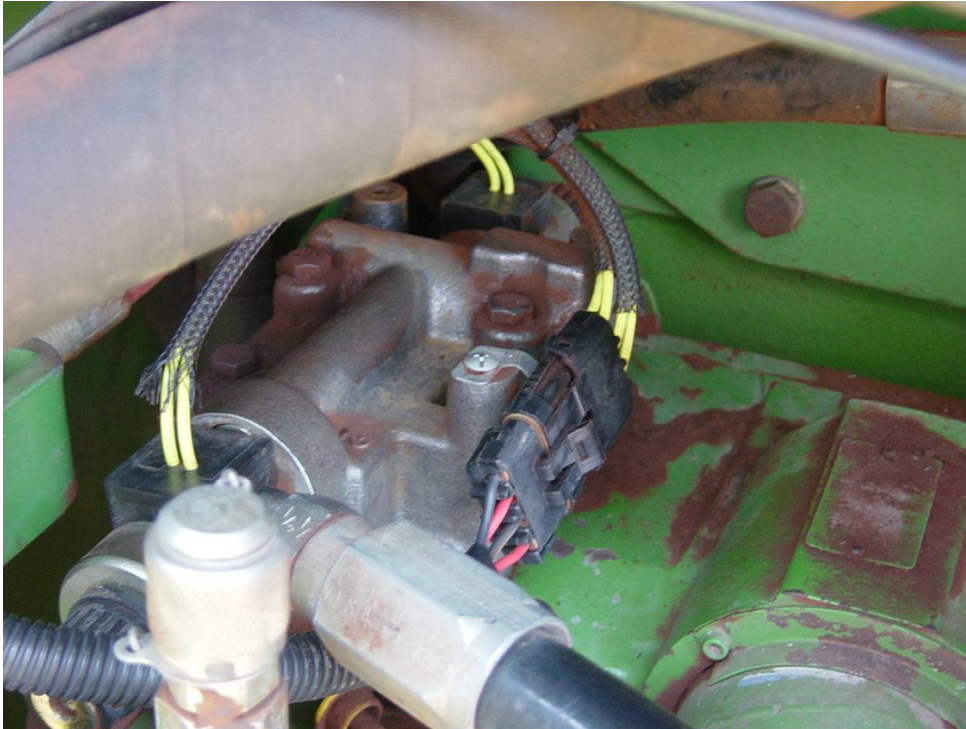
Figure 50 Eaton electro-hydraulic proportional pump controller fitted to the experimental harvester
