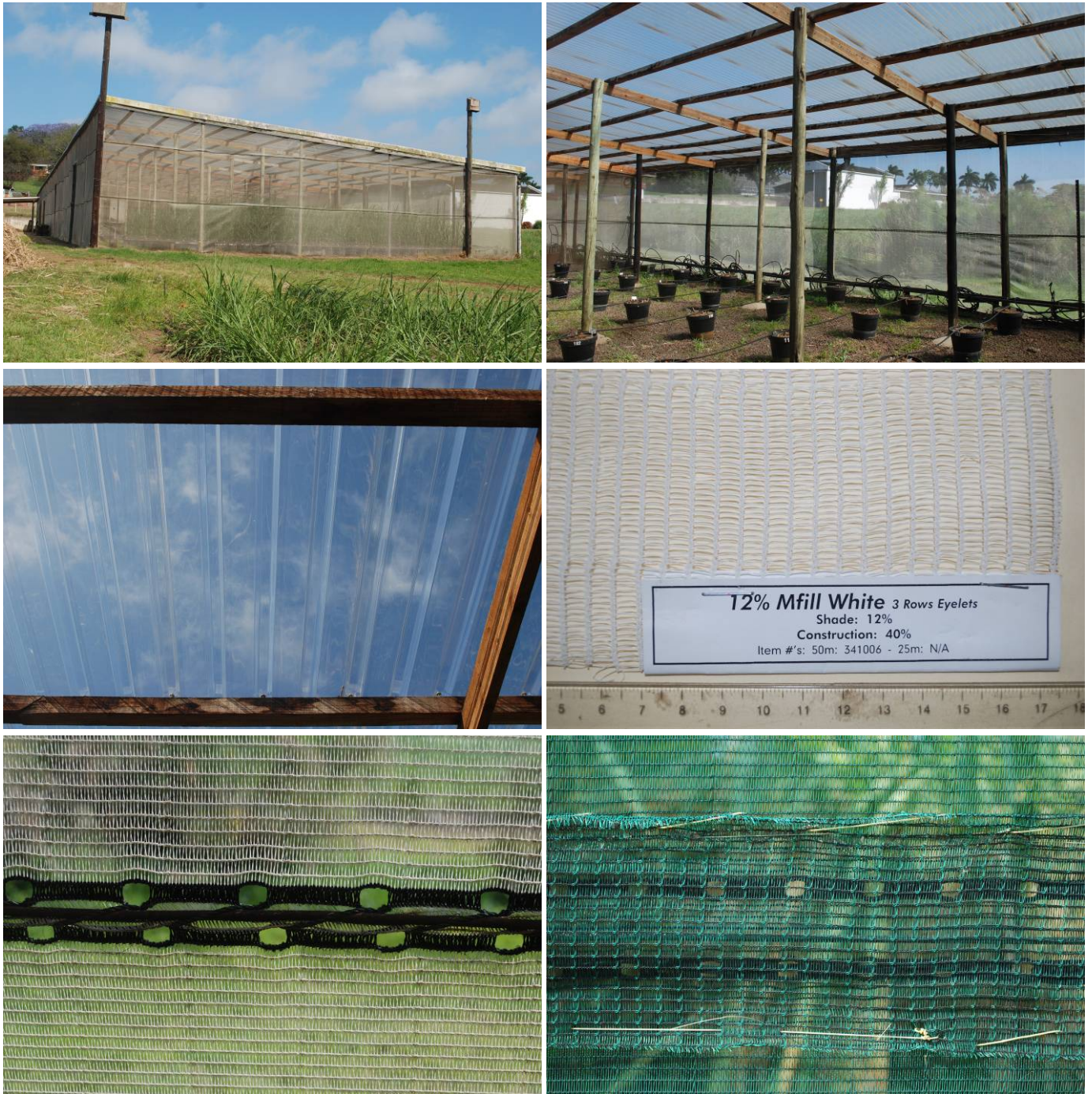
Figure 1 - Shadehouse at SASRI: top, external and internal view; centre, roof material (clear polycarbonate) and wall material (shadecloth); bottom, horizontal joining of cloth panels and early attempt to improve insect-proofing by covering joint with second layer of cloth
