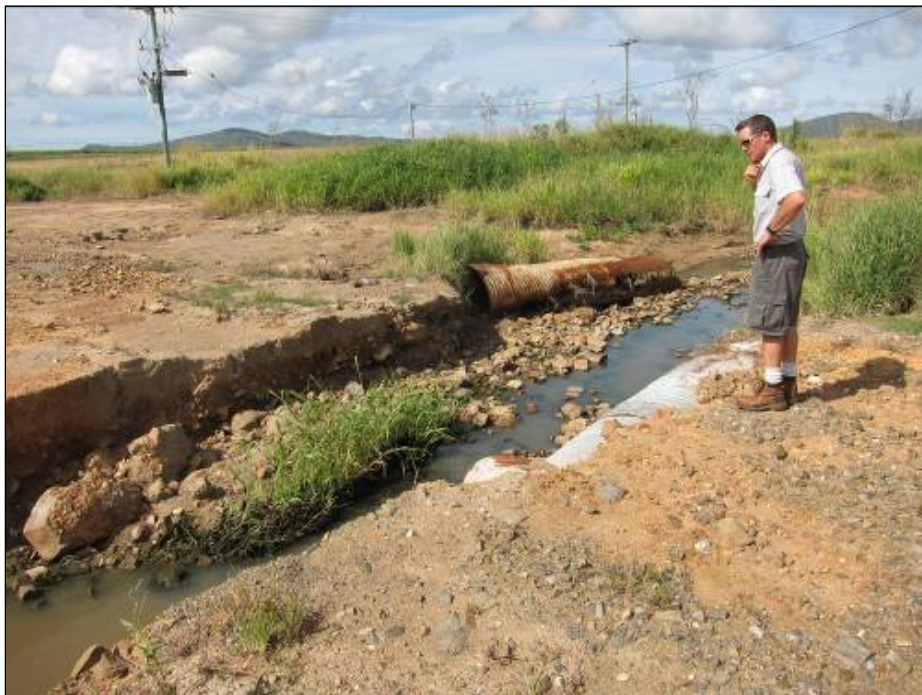
21 Feb 2011 - One of the road crossing washouts on a cane farm caused by heavy rain
