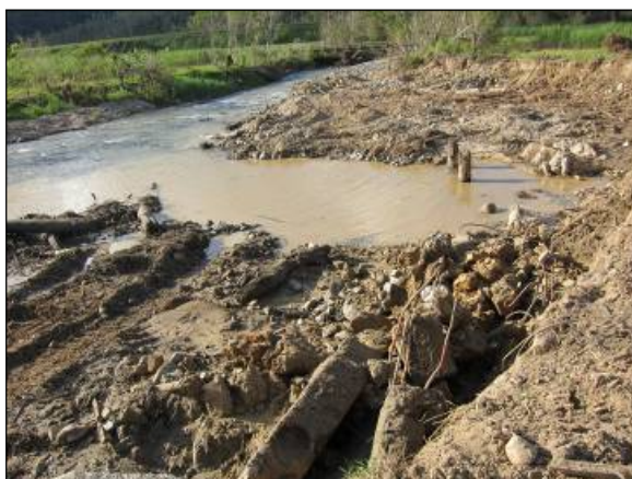
22 Feb 2011 – Missing tram line bridge, Number 3 Branch, Liverpool Creek
