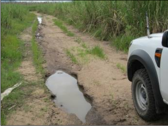
23 Feb 2011 - Washed out headland, Warrami
