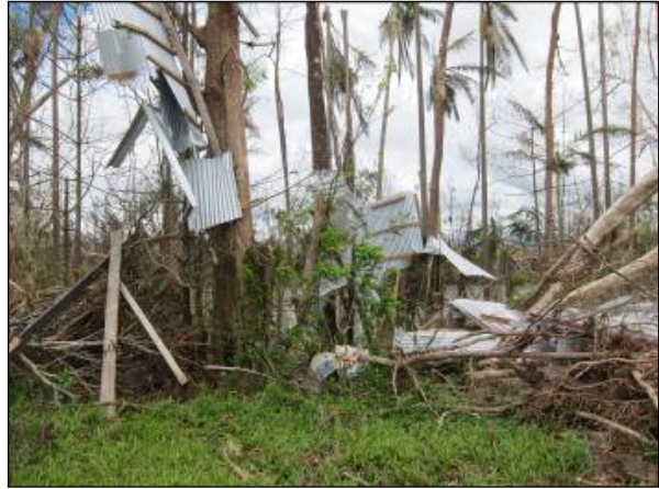
23 Feb 2011 - Destroyed farm building between Tully & Tully Heads
