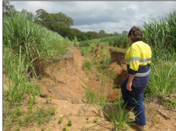
4 Mar 2011 – Major washout of farm road, Carmila West
