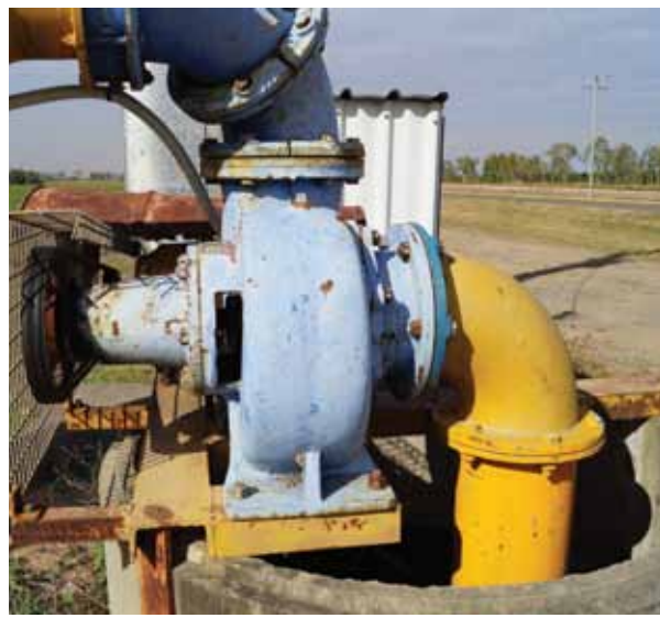
Left: Furrow irrigation. Center: Centrifugal pump on a well. Right: Poorly performing pumps have high electricity costs.
