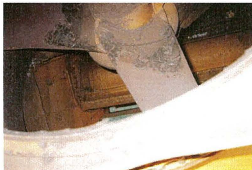
Image 2 - View of fan assembly of secondary extractor. The trash flow through the fan absorbs considerable power, reduces the aerodynamic efficiency of the fan and caused accelerated wear.
