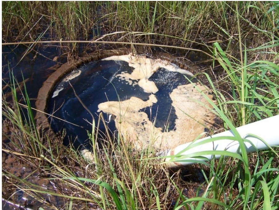
Figure 10. Overflow well into which the wetland Bay 6 discharges. A pipe under the western bund wall connects this flow back into the North/South farm Discharge Drain. White PVC pipe is access for water quality monitors.
