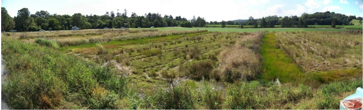
Figure 4. Panoramic eastward view of wetland middle bays 3, 4, and 5 (from left). Bays 1 and 2 cannot be identified at the extreme left, on this side of the highway. In the foreground is the overflow weir (# 4) through the bund wall between Bays 4 and 5 along with its “borrow-pit” vegetated with Eleocharis reeds.
