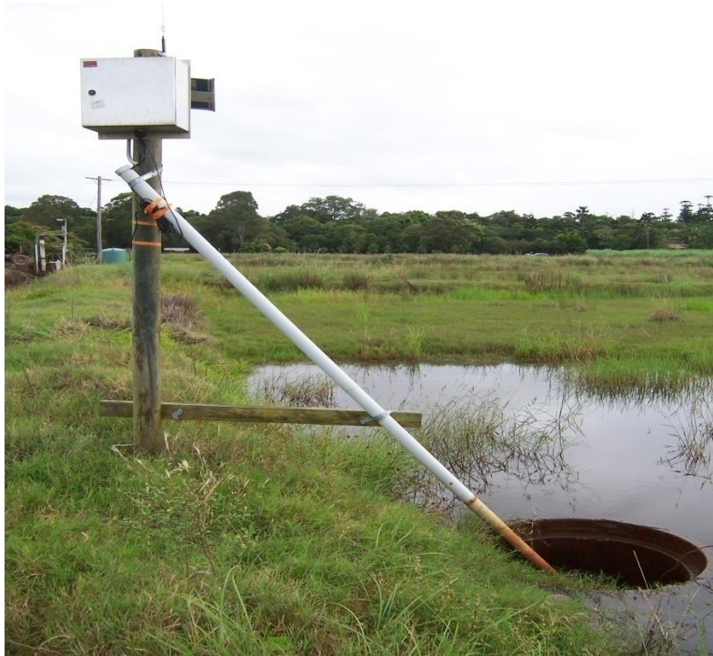
Figure 11. Bay 6 overflow well with water quality monitoring unit.
