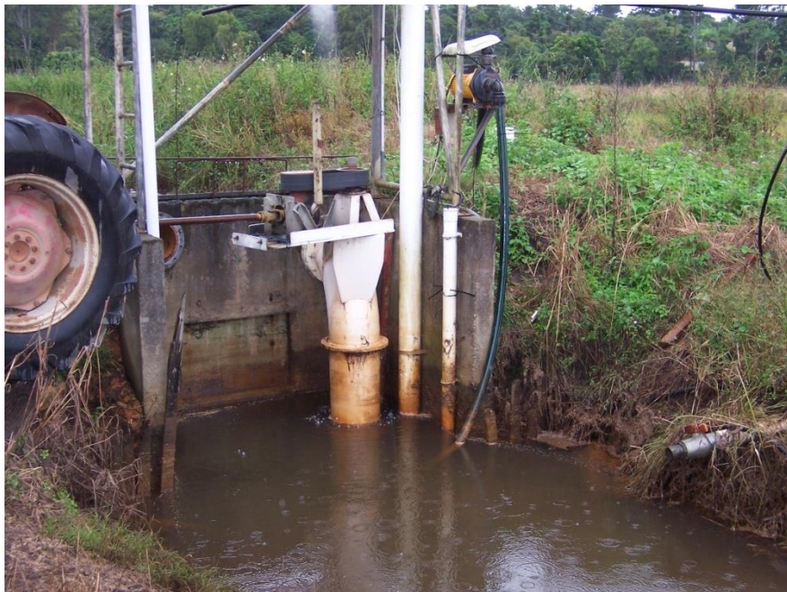
Figure 8. Small yellow electric pump supplying input to wetland. Main farm drainage export by PTO pump while large electrical pump temporarily under repair.
