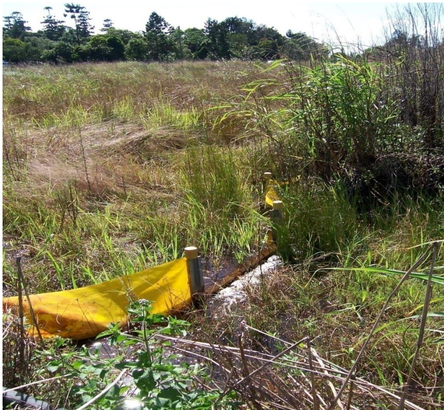
Figure 5. Detail of overflow weir # 4 between Bays 4 and 5.
