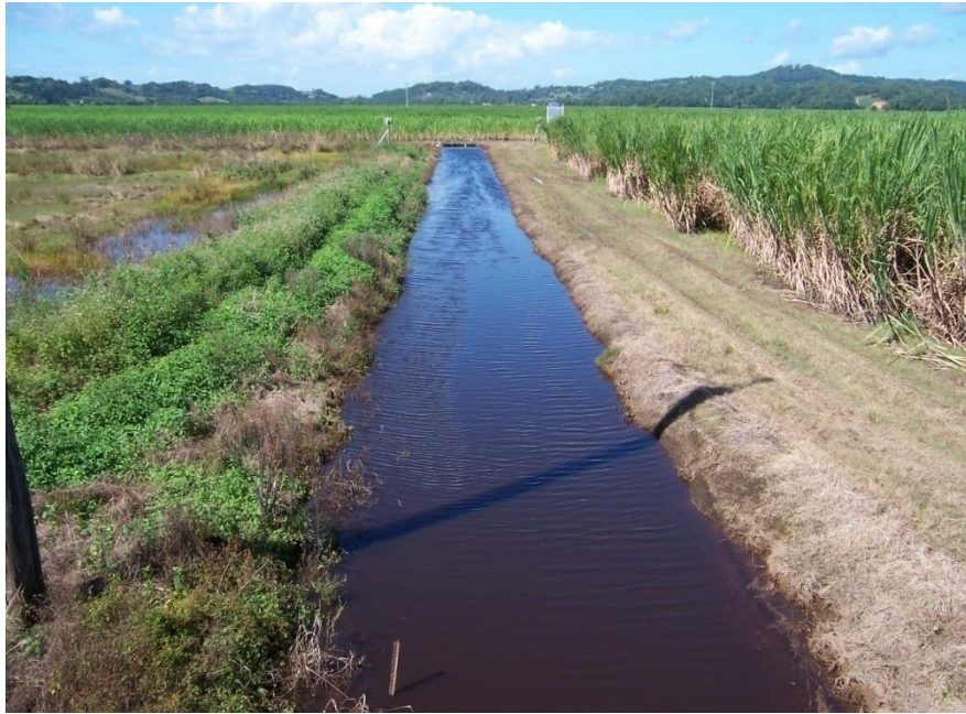
Figure 7. Upstream southward view of farm's Discharge Drain from which water is pumped into the wetland. The monitoring unit at the wetland outlet well is in the distant LHS.
