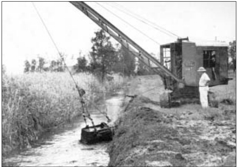
Figure 1. A floodplain drain being cleaned using a dragline excavator. (Photo: NSW Sugar Milling Cooperative)
