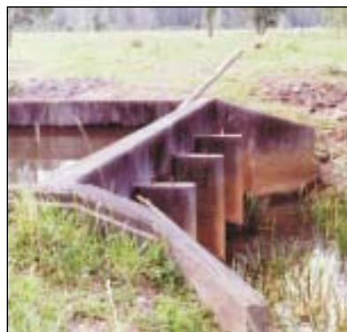
Figure 6. Floodwaters (centre left) are prevented from filling a natural backswamp by floodgates. Floodgates and flood mitigation works have helped reduce the frequency and severity of coastal flooding.
