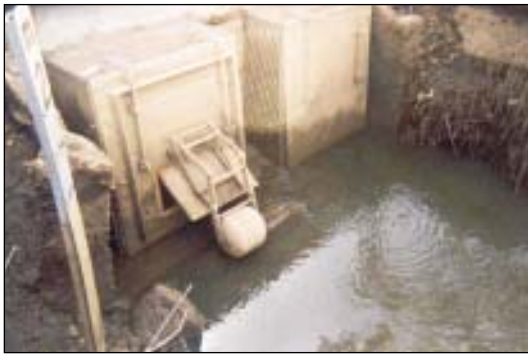
Figure 21. Tidal floodgates. As the tide rises the float lifts and automatically closes the gate, which then seals tight due to water pressure. (Photo: Frederieke Kroon)
