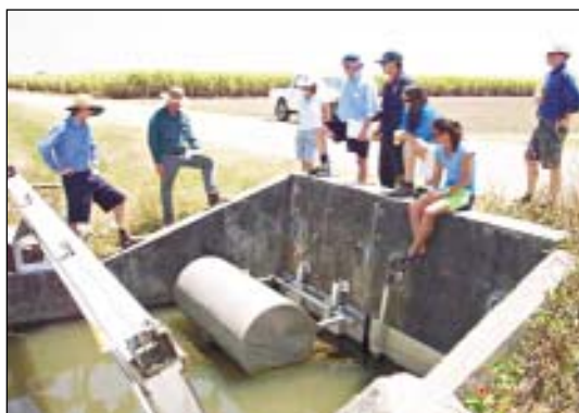
Figure 55: Inspecting a tidal floodgate on a drain in the Clarence River. A cooperative attitude between all stakeholders and a willingness to learn and exchange information are important features of all successful projects. (Photo: Rob Lloyd)
