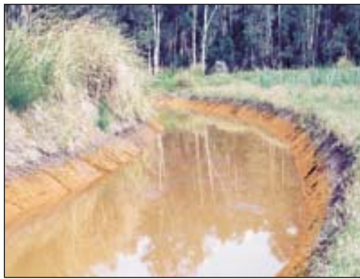
Figure 29. Bright orange iron staining along the sides of a drain – an indicator of chronic acid conditions.
