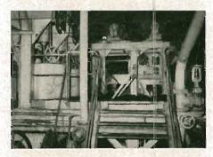
The low-grade fugal station at Farleigh Mill.
