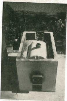
Soil sterilizing boiler. These are used at all stations for sterilizing seedling flats.
