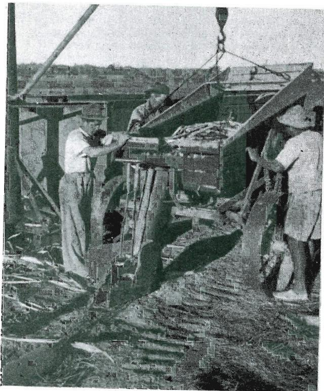
FIG. 8.—Large dipping plant, showing the planter-box full of dipped setts being lowered into place on the planter-frame.
