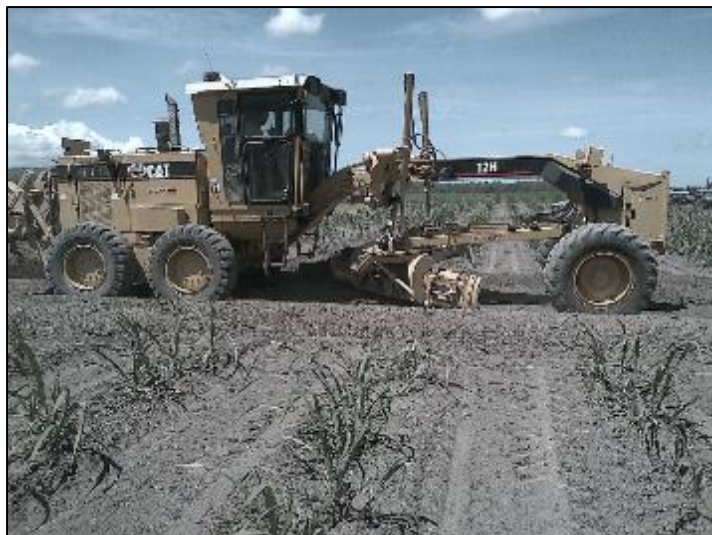
Figure 5.4 Earthworks in order to bund plots for waterlogging treatments.
