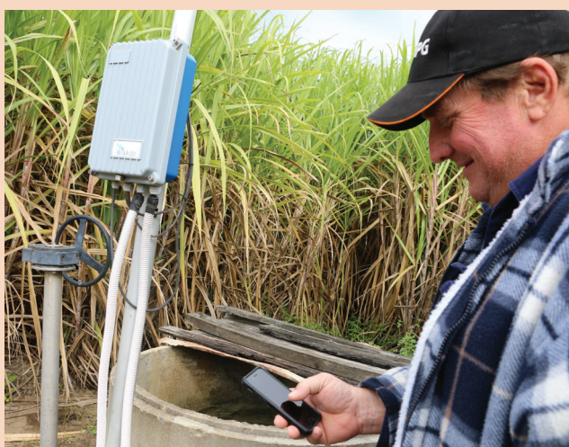
Above: Denis Pozzebon operating his automated furrow irrigation system.
