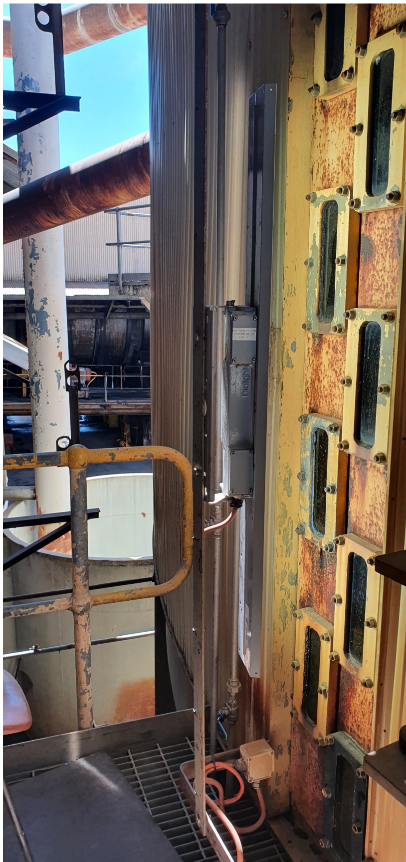
Figure 5 Clarifier at Victoria Mill before the visual camera system installation
