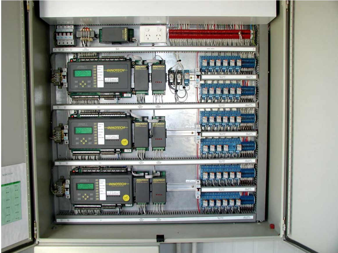
Figure 3: Direct digital controller board
