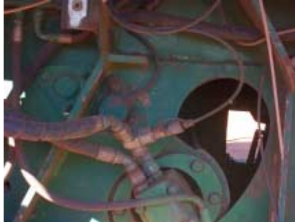
Figure 12 - Feed roller displacement sensor and pilot tube arrangement
